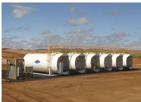
The tanks are generally, steel single wall, steel/steel double wall, steel/fibreglass double wall, in the case of the double wall, the design is industry and regulator compliant and certificated to international standards. The uniqueness of the design is that there is full material and manufacture traceability and uniquely the gap between the primary tank wall and the secondary tank wall is supplied to the customer with a vacuum and this vacuum forms a monitoring mechanism for the future and
