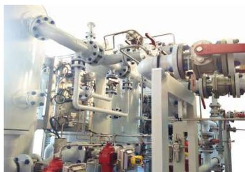
Examples of pipe spools with in various packages demonstrating the accuracy achieved in flange to flange connection over multiples of length and orientation.
